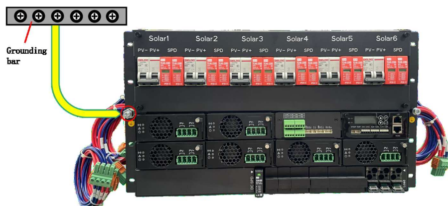
Figure 1-2 Installing a protective ground cable
